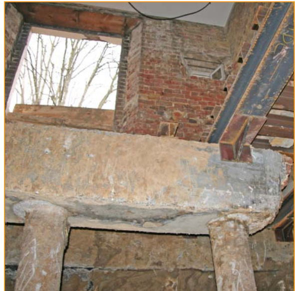
Exposed temporary works pile
